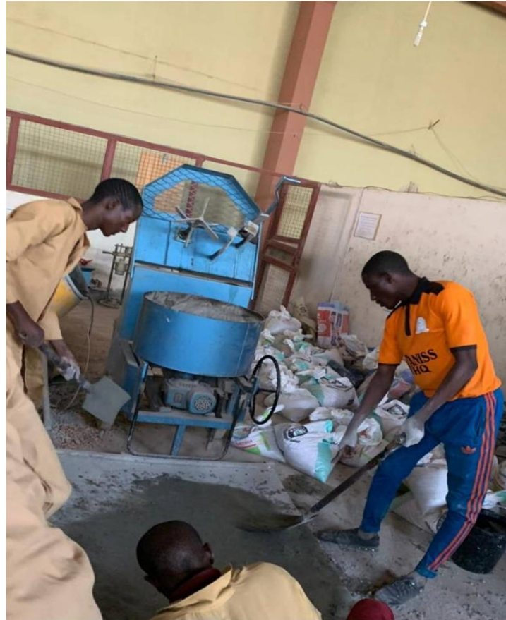
Fig. 5. Mixing of concrete constituents.
