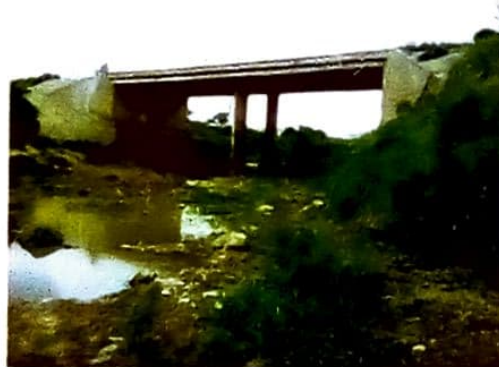
Figure 2 Kpakungu bridge spanning the stream
