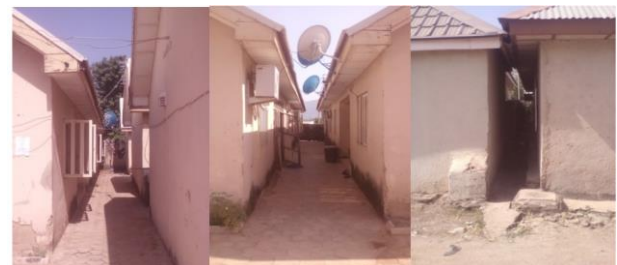
Figure 3. Windows of houses opening into a narrow lobby with insufficient setbacks between buildings, causing insufficient airflow for adequate ventilation.
