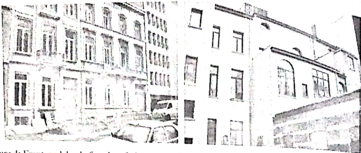
Figure 4: Front and back façade of the renewable energy house, Brussels, after refurbishment. Source: Adapted from New4Old [27].
