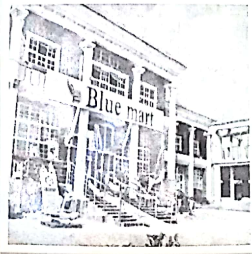
Plate 4: Showing the use of deep verandah to shade the windows at Blue Mart Minna
