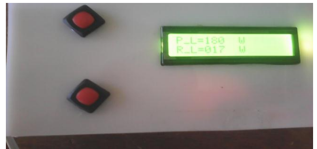
PLATE III: PROJECT SHOWING CIRCUIT BREAKER WITH MAX VALUE OF POWER ALLOWED AND CURRENT POWER CONNECTED.
