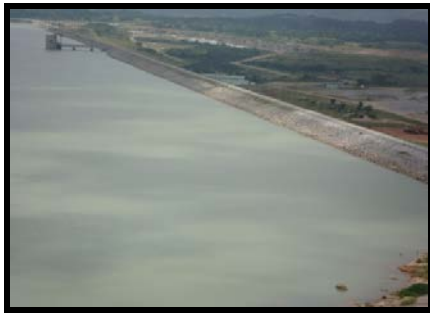
Plate I. Over View of the Gurara Dam Intake with Tower at Extreme Left
