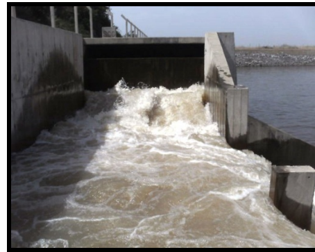
Plate IV. The Outlet Structure where the Water from Gurara Dam enters the Lower Usuma Dam during full discharge
