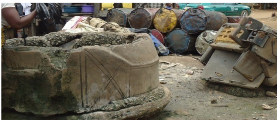
Plate 1. Poor on-site sanitation around a hand-dug well at Erena
