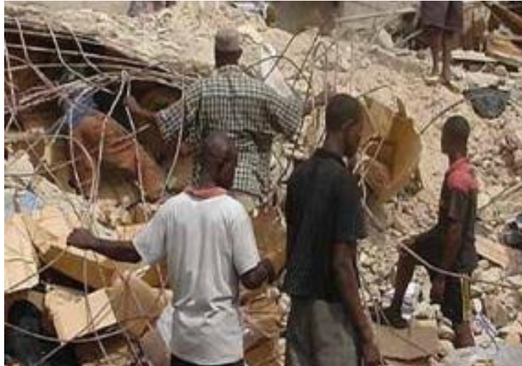
Figure 1. A collapse building due to use of sub-standard material (Source: Author, 2012)
