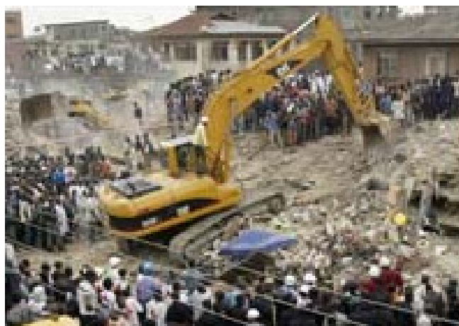
Figure 2. Collapsed building arising from foundation failure (Source: Author, 2012)
