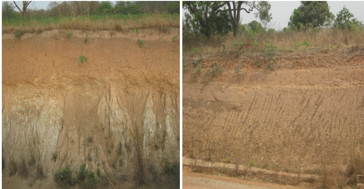
Plate 1 and 2: Typical Matured Laterite Profiles Along Road Cuts (L6SP3 & L1SP1)
