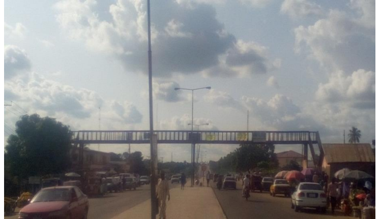
Plate VIII: A Pedestrian Overhead Bridge on the Bosso Road
