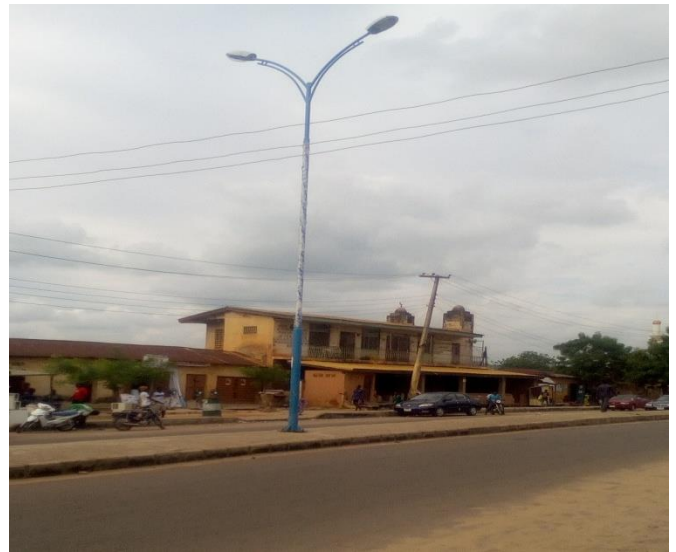
Plate VI Electricity Powered Street Light along Old Airport Road
