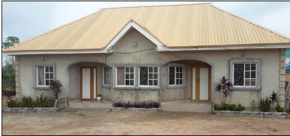
Plate XI: 2-Bedroom Semi detached Modern residential House in Minna, Niger State (North Central Nigeria). Source: Author's fieldwork (2015).
