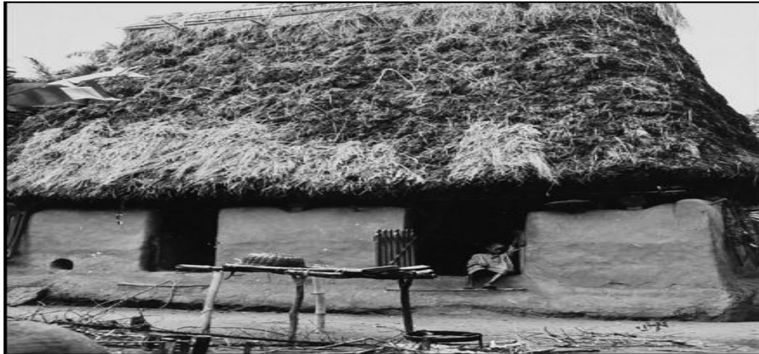
Plate I: Traditional Building in Anambra State, Showing Thatch-roof on Load-bearing wall system. Source: Tropenmuseum, 1967.
