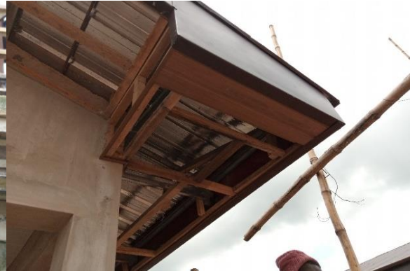
Fig 2: Conventional Roof Wooden Eave Fascia.
