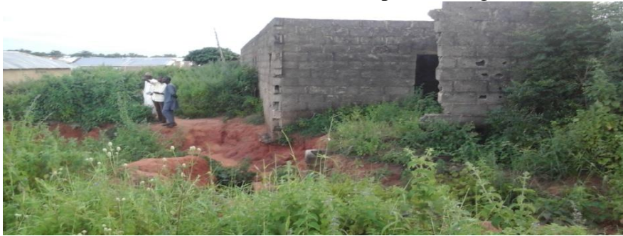
Figure 3: an abandoned structure beside an excavation pit with some collapsed parts in Dikobororo area
