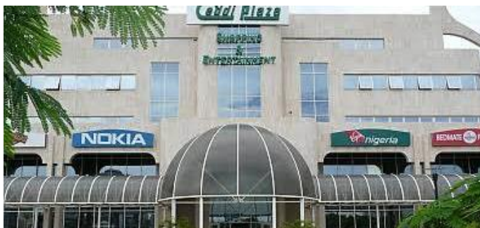
Plate II: Windows and Surveillance Source: Author`s field work (2020)
