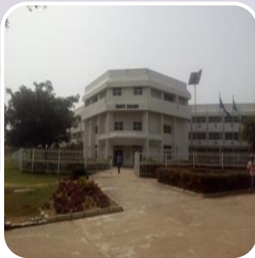
Plate I: Administrative building, Federal University of Technology, Minna. (B1)
