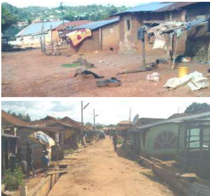
Plate 2: Building Types at Oworo Community and at the Periphery of Felele Town
