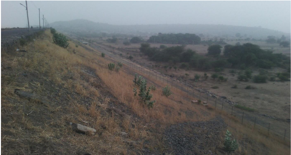
Figure 2: Downstream face of the dam (Source: Self picture snap)
