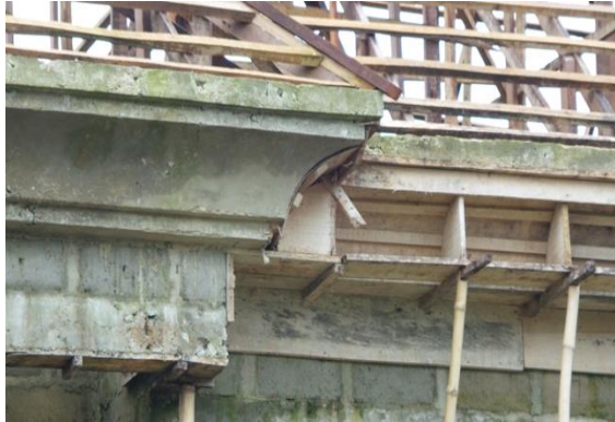
Fig. 1: Roof Concrete Eave Fascia. Source: Author's fieldwork
