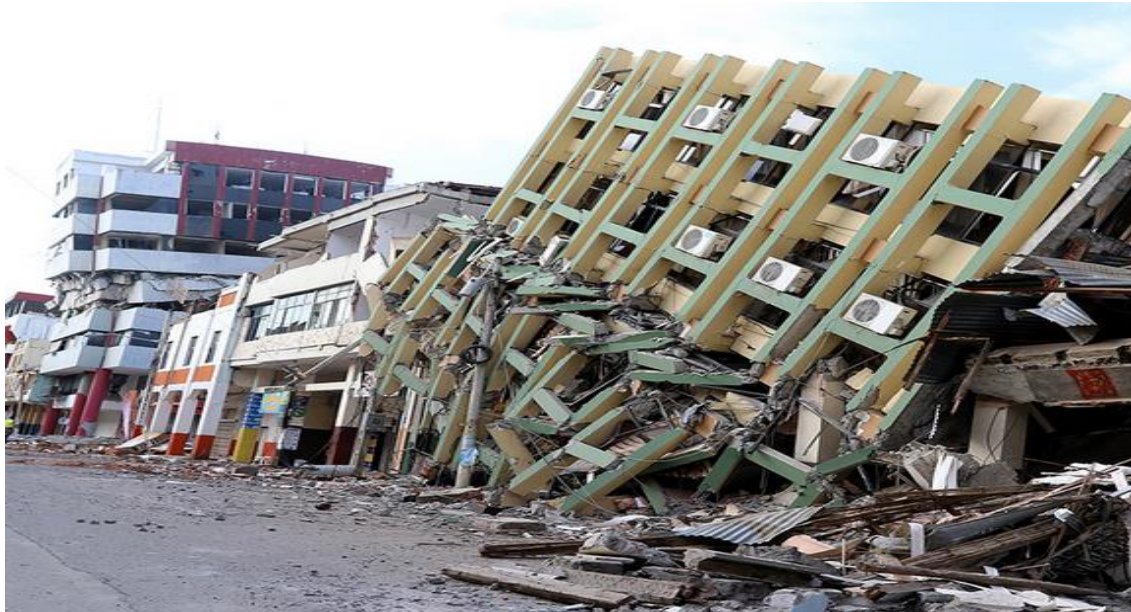
Figure 1 Ecuador earthquake, 2016 after a 7.7 magnitude. Source: P, Brannen 2016.
