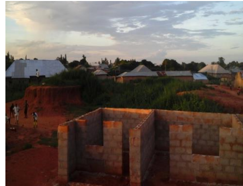
Figure 3: A building under construction In an excavation pit Dikobororo ward 2
