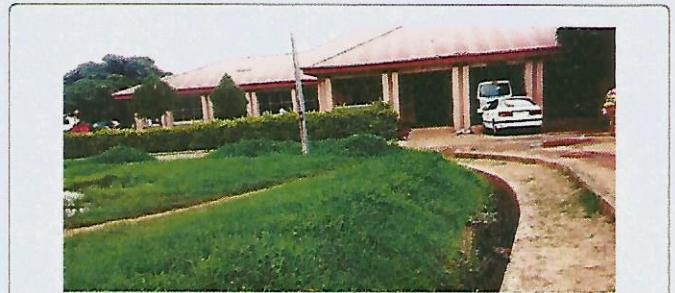
Figure 3: Plate III-Gwamna Awon general hospital Nasarawa road, Kaduna administrative block.
