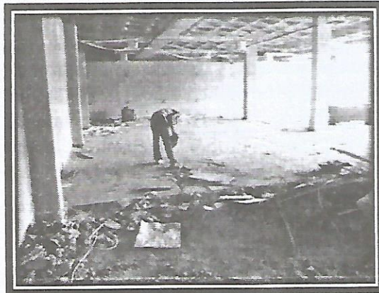
Plate 1: Removal of Floor Finish using powered tools
