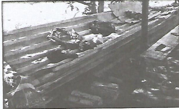
Plate 3: Roofing sheets carefully salvaged.
