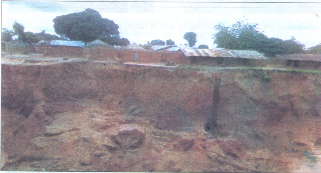
Figure 4. Parts of those houses that are more vulnerable to severe gully erosion.
