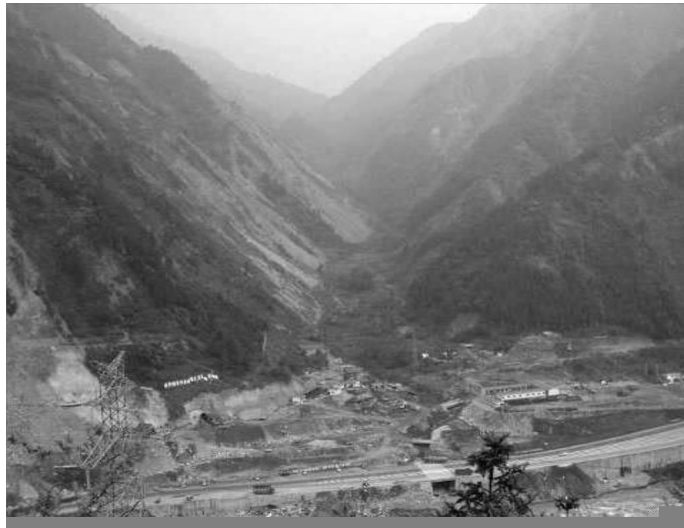
Figure 4: Steep Slopes that Aided Movement of Materials During the Yingxiu Landslide
